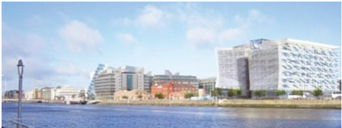
Bank's New Headquarters, North Wall Quay, Dublin 1.
